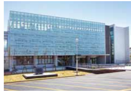
The Exterior of the Library
