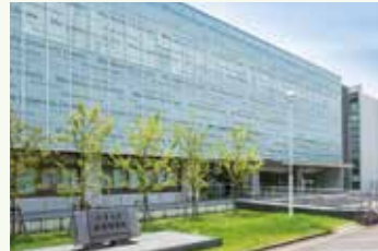
The Exterior of the Library
